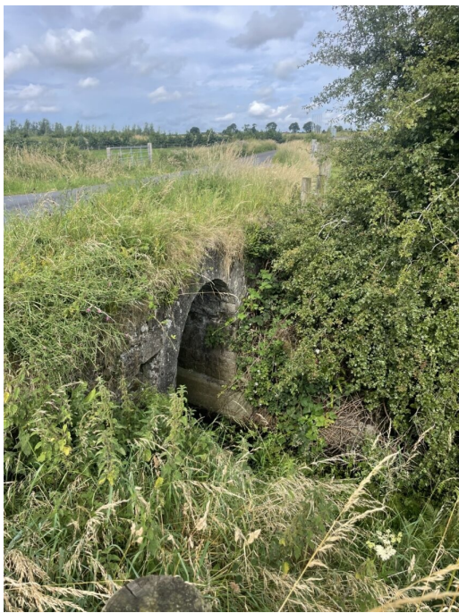
Looking Northeast, Facing Upstream
