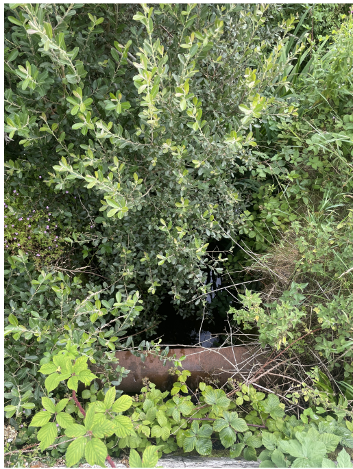
Looking East, Facing Upstream
